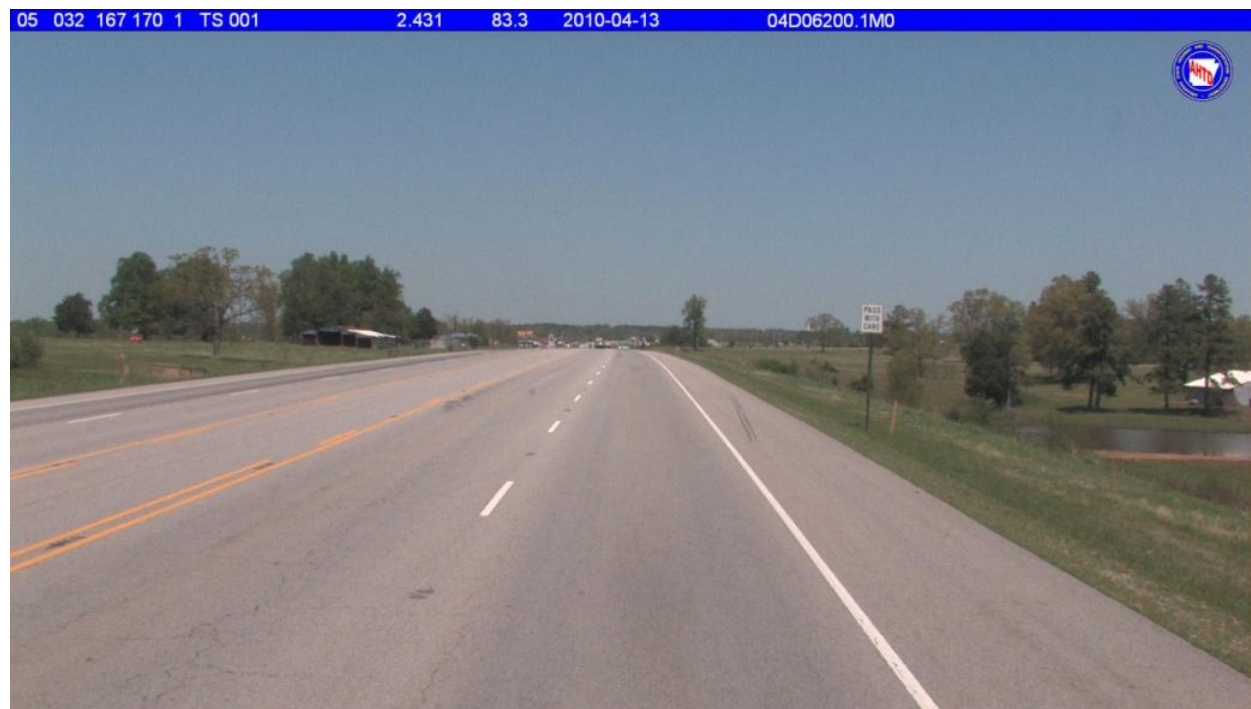
Figure 6.23 ROW of R50084 in April 2010
