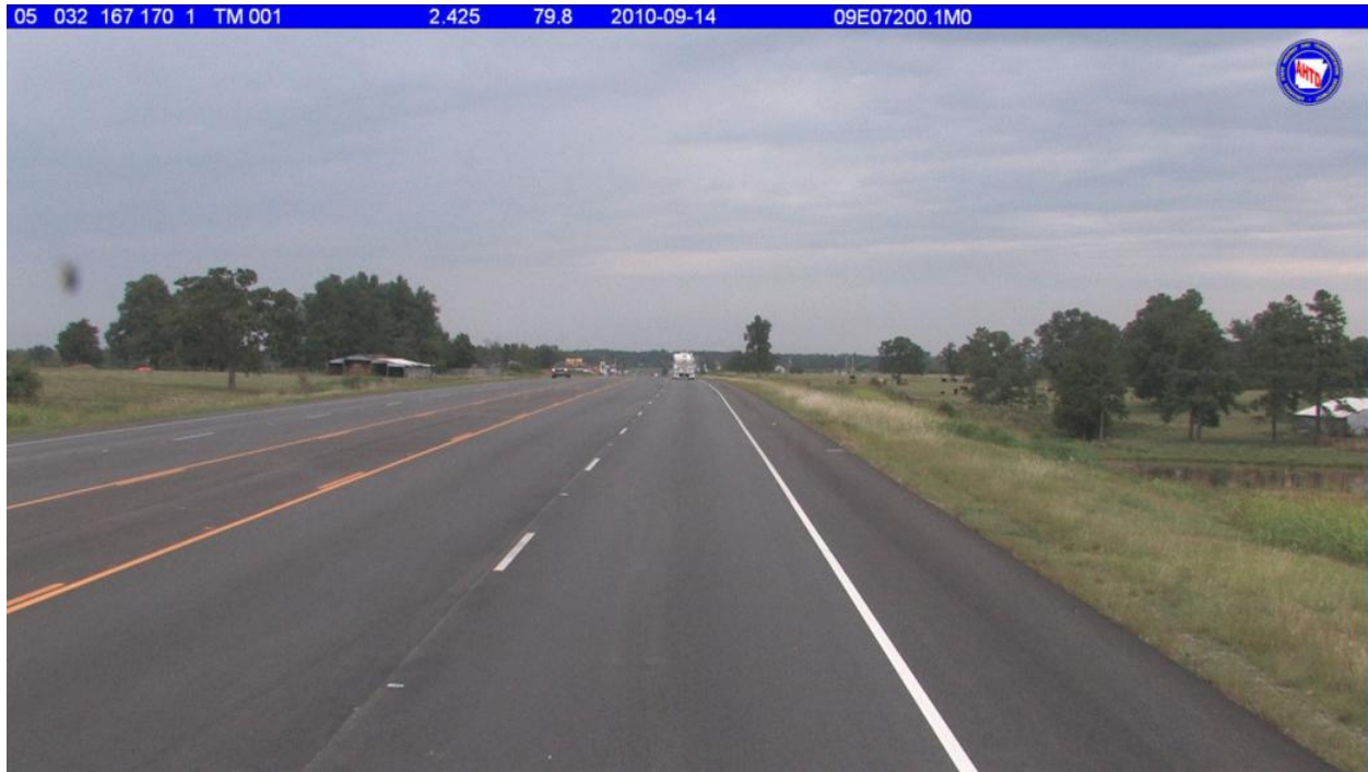
Figure 6.24 ROW of R50084 after resurfacing in September 2010
